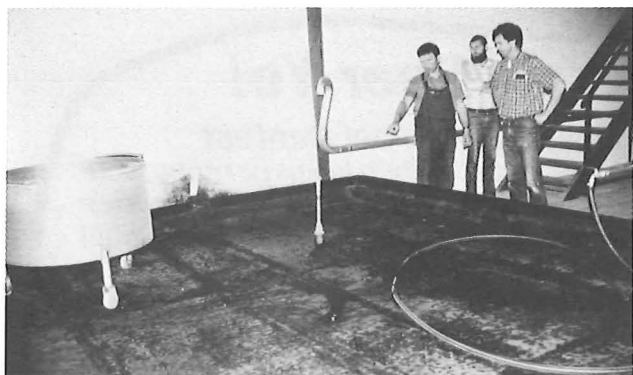
Brewmaster Hans Senger of Brauerei Barth explains the function of the cool ship, a shallow pan where beer is air-cooled before forced chilling.
